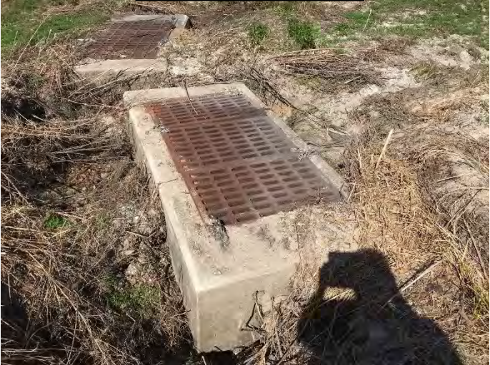
Pond Structure 70-1 in foreground
